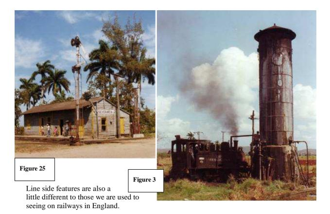
Figure 35 shows the station at Persiverancia, typical of most small rural stations throughout Cuba. The only unusual item is the double signal protecting the diamond crossing in front of the station. Figure 36 is a view of the unusual water tower at Ruben Martinez Villena mill, watering the only coal-fired engine encountered in Cuba. This is number 1207, a 2-4-0T built by Henshel in Germany in 1912.
